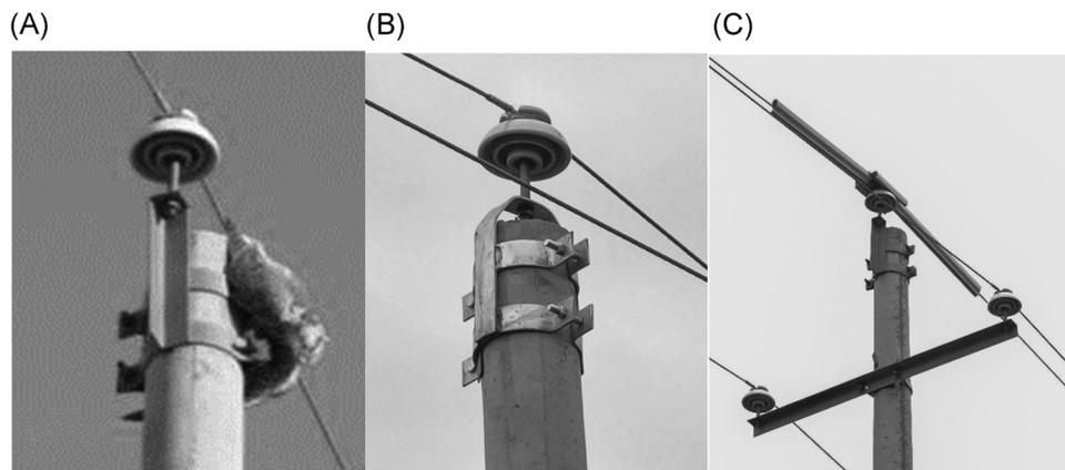
**Figure 1.** Pole top configurations at the Munkhkhayan-Uulbayan 15 kV electricity distribution line, Sukhbaatar Province, Mongolia in 2013. (A) Standard vertical mount (control) and (B) arch-type mount for pin insulator at phase 1 on top of tangent poles. (C) Insulation cap and covers fitted on phase-1 pin-insulator and conductor cables (P1 covers). Electrocuted Saker Falcon shown in A.
