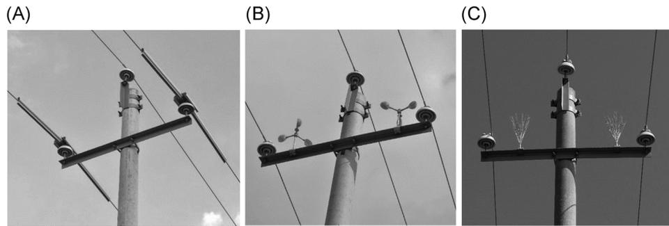
**Figure 2.** Crossarm configurations at the Munkhkhaan-Uulbayan 15 kV electricity distribution line, Sukhbaatar Province, Mongolia in 2013. (A) Insulation cap and covers fitted on the phase-2 and -3 pin-insulators and conductor cables (P2/3 covers). (B) Rotating mirror perch deterrents fitted to the cross-arm adjacent to the phase-2 and -3 pin insulators (mirrors). (C) Brush perch deflectors fitted to the cross-arm adjacent to the phase-2 and -3 pin insulators (deflectors).
