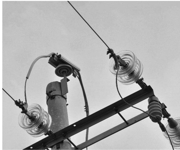
**Figure 3.** Configuration of jumper wires at anchor poles at the Munkhkhaan-Uulbayan 15 kV electricity distribution line, Sukhbaatar Province, Mongolia in 2013. Pin insulator cover and flexible hose insulation on jumper wire at phase 1 of an anchor pole, where the jumper wires for phases 2 and 3 had been reconfigured to pass under the cross-arm via a suspended insulator.
