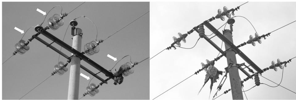
**Fig. 1.** Left: anchor pole with jumper wires (arrowed) over the crossarm at phases 2 and 3 (3-over anchor pole). Saker Falcon electrocuted at 3rd phase jumper wire. Right: reconfigured anchor pole with jumper wires passing under the crossarm at phases 2 and 3 (1-over anchor pole). Upland Buzzard electrocuted at 1st phase jumper wire.
