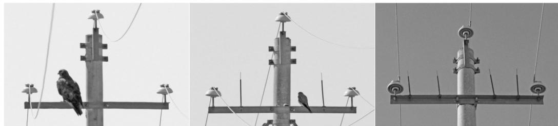
**Fig. 2.** Left: Upland Buzzard perched on line pole crossarm with 0 perch deflector spikes. Centre: Common Kestrel perched on line pole crossarm with 2 perch deflector spikes. Right: line pole crossarm with 4 perch deflector spikes.
