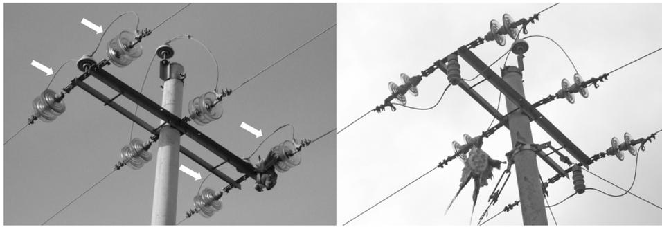
**Fig. 1.** Left: anchor pole with jumper wires (arrowed) over the crossarm at phases 2 and 3 (3-over anchor pole). Saker Falcon electrocuted at 3rd phase jumper wire. Right: reconfigured anchor pole with jumper wires passing under the crossarm at phases 2 and 3 (1-over anchor pole). Upland Buzzard electrocuted at 1st phase jumper wire.
